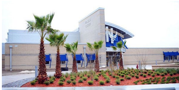
Figure 9. Green building. Cool-roof technology and a solar-generated hot water system are expected to help produce energy savings of 9 percent at the new fitness center at Tyndall AFB, Florida. (US Air Force photo, accessed 6 February 2012, http://www.af.mil/shared/media/photodb/photos/100513-F-1234E-102.jpg )
