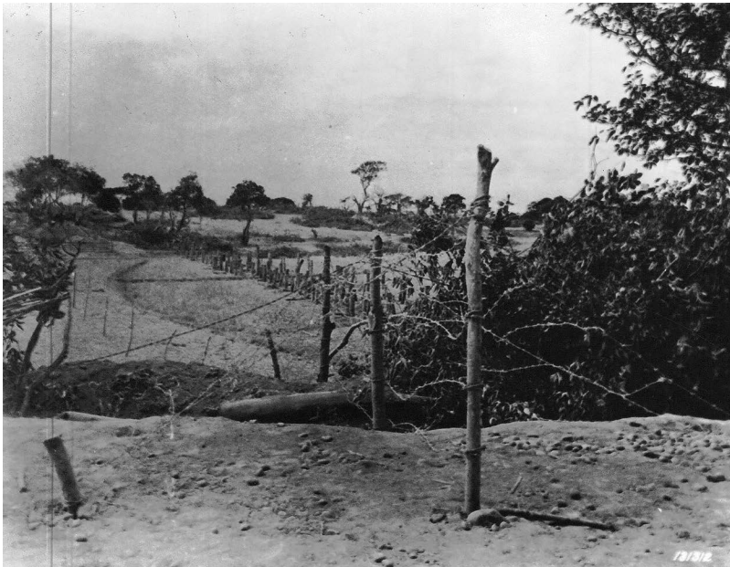
Pile-type tank obstacles with double-apron barbed wire fencing, Bataan, 18 January 1942
